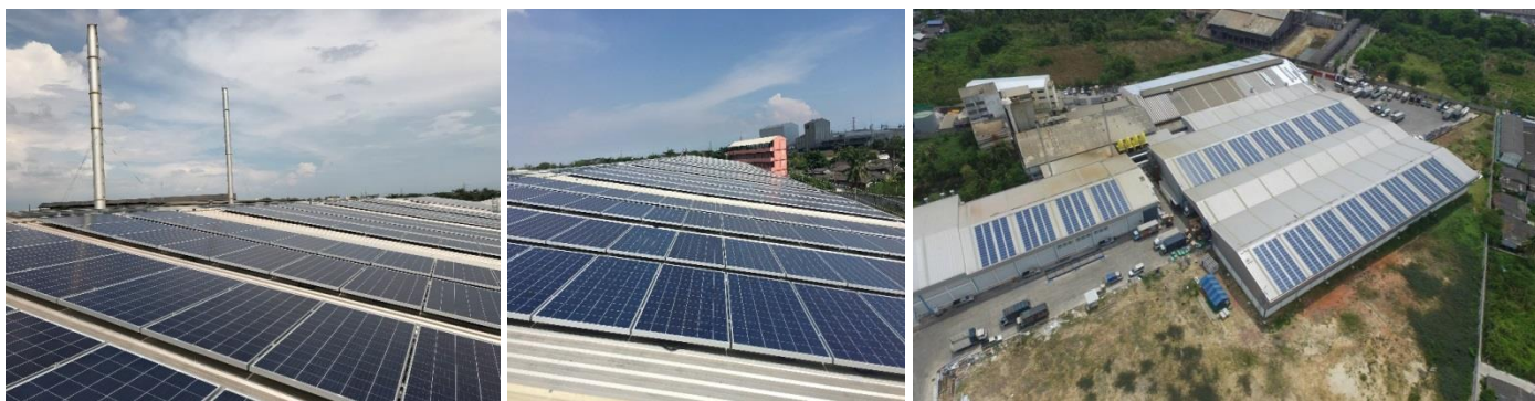
Figure 2 : The construction of SNNP solar roof project with 384 KW capacity
