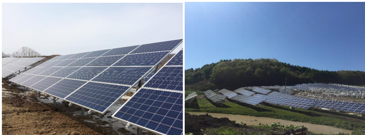
Figure 3: The construction of Hidaka project with 17 MW contracted capacity in Japan
